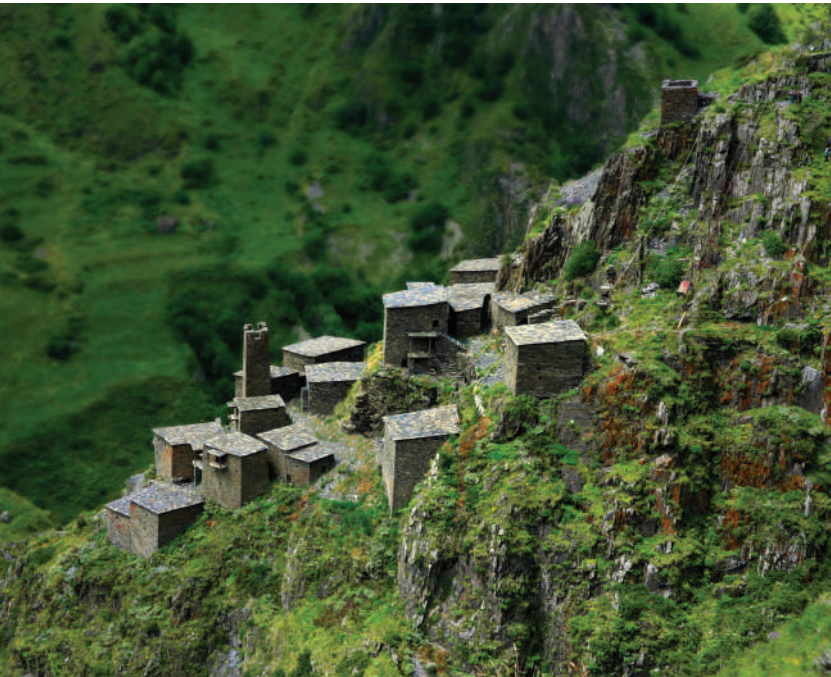
10 The recently renovated Village Mutso in Khevsureti
